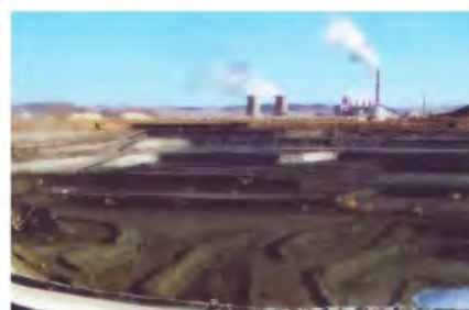
Shenhua Group Shendong Daliuta Wudangou Coal Project
