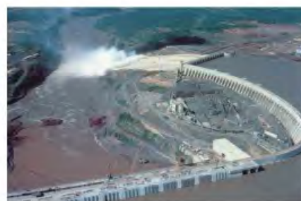
Three Gorges Hydroelectric Power Station
