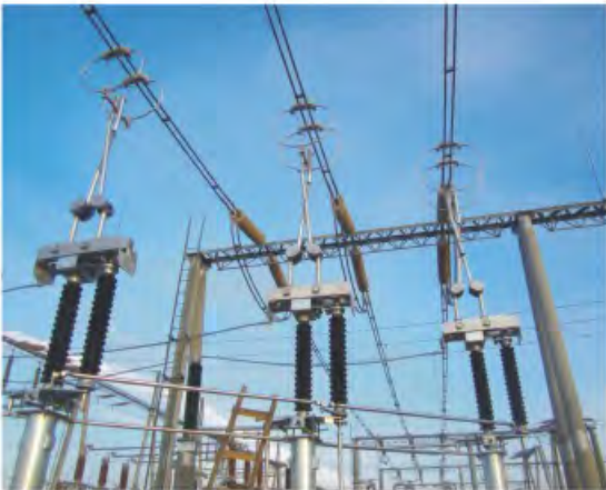
Pantograph Disconnector (126kV-550kV)
