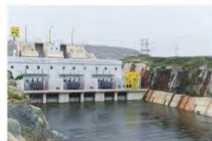
Cote d'Ivoire Subley Hydroelectric Power Station
