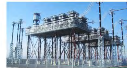
The Jindongnan-Nanyang-Jingmen UHV AC transmission project 1000kV Changzhi Substation, Series Compensation capacity: 1503 MVAR Client: State Grid Corporation of China
