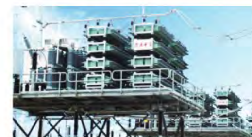
Guangxi Hezhou 500kV Substation Serial Compensation Capacitor Bank
